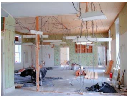
The RCA/Marconi Operations building is gutted and ready for renovation and new exhibits.
